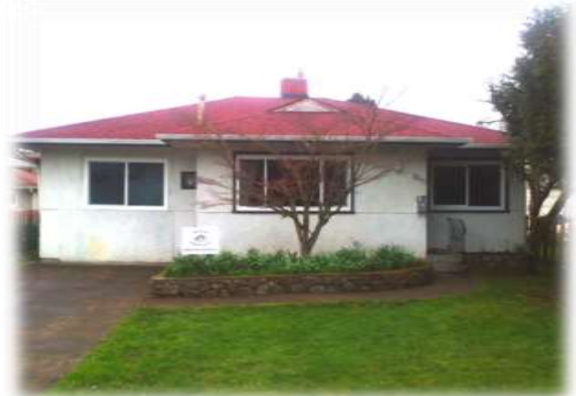
Shelbourne Community Kitchen's New Location 3541 Shelbourne Street between Cedar Avenue and Donnelly Avenue
