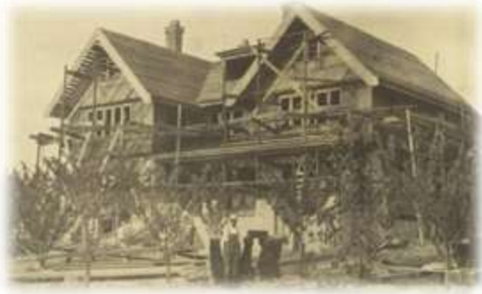
1140 Tattersall Drive under construction
