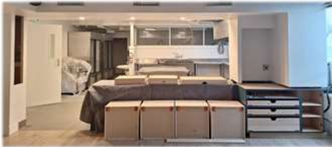
New cabinets to go into the kitchen
