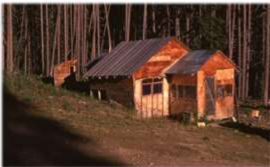
The cabin on Whipsaw Creek
